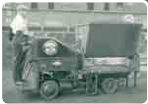
CLARK introduces the world's first Internal-Combustion platform lift truck. The Truclift is the first industrial truck to use hydraulic power to lift a load.
